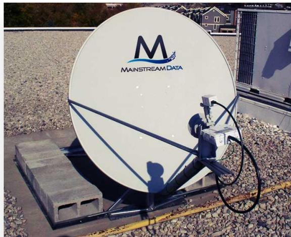
1.2M antenna with non-penetrating roof mount
